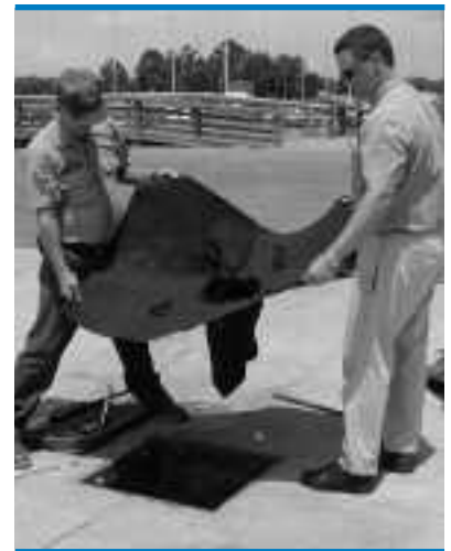
Inlet filter slip being installed.
