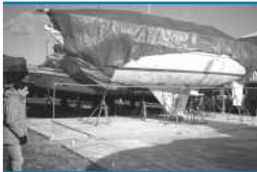
Concrete work pads are raised and surrounded by permeable gravel to control runoff.
