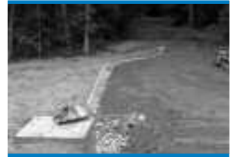
Level spreader constructed of concrete.
