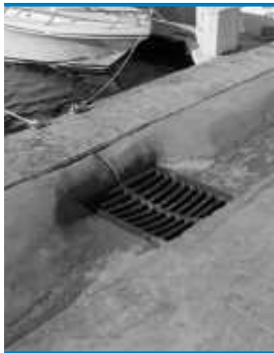
Stormwater inlet draining directly to marina basin.
