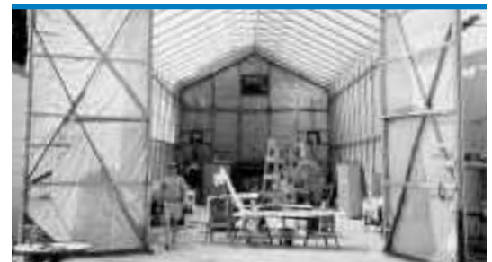
Temporary work enclosure located on Shelter Island, New York.
