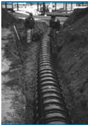
Infiltration chambers being installed.
