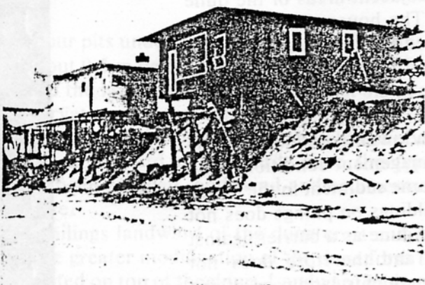
FIGURE 7. Condition of the dune beneath houses elevated on pilings after passage of the storm of February 7, 1978.
