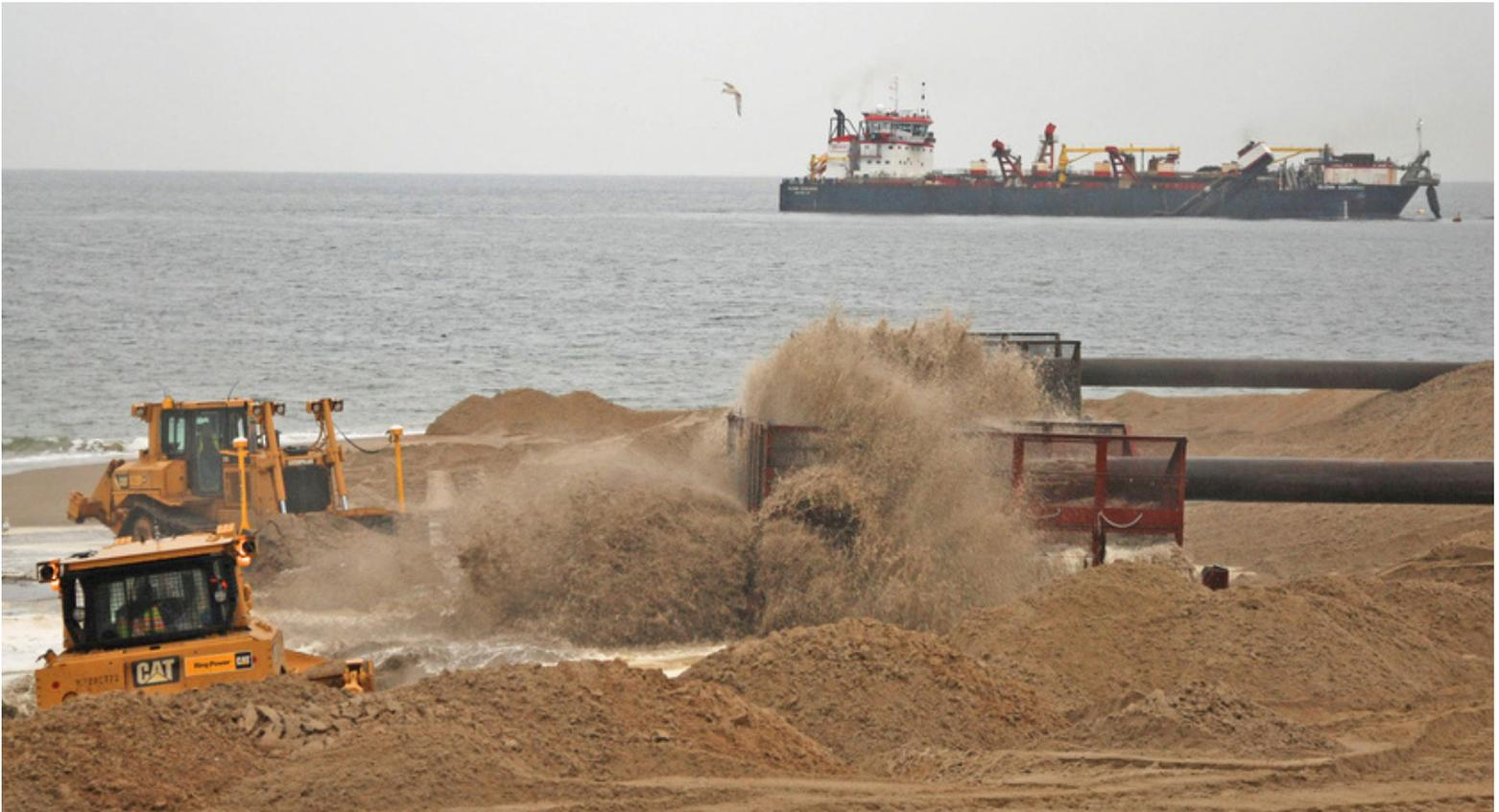
*During beach nourishment, an offshore supply of sand is pumped by a dredge onto the beach where bulldozers reshape the sediment. Image credit: US Army Corps of Engineers*
