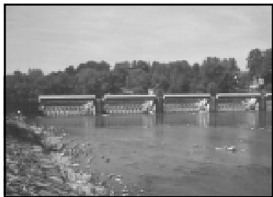
The Caughdenoy Dam's gates on the Oneida River.
