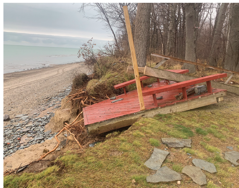
[Figure 2] Seiche-event shoreline damage submitted to New York Sea Grant from a property owner in Irving, NY. Waves produced by this seiche eroded the loose sediment above shale bedrock, undermining coastal structures and uprooting trees. Photo submitted through New York Sea Grant Virtual Site Visit form.
