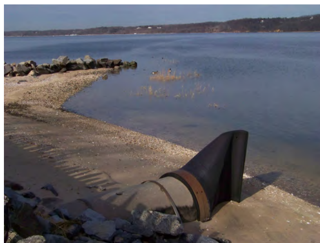
Stormwater mitigation projects protect water quality.
