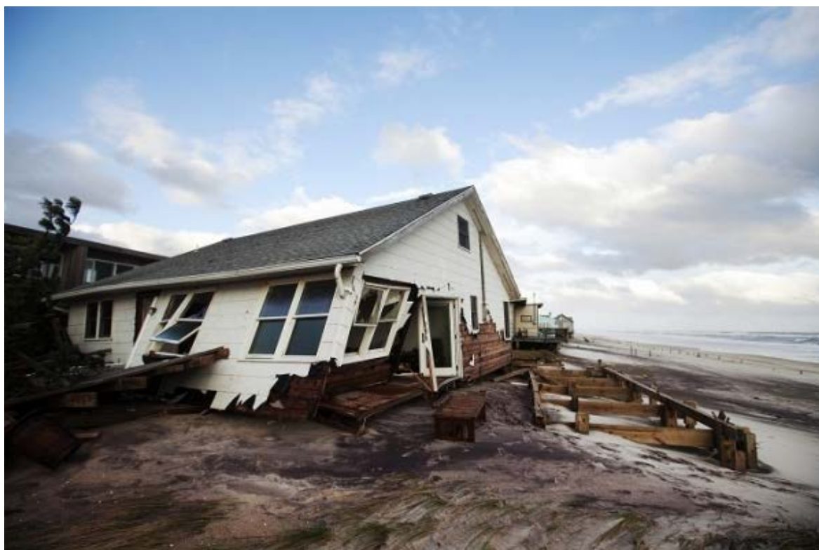
Damaged house is seen after Hurricane Sandy passed through in the greatly affected community of Atlantique on Fire Island, New York.(Photo : Reuters)
