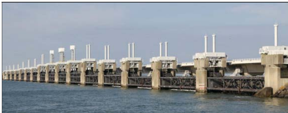
Floodgates in the Netherlands
