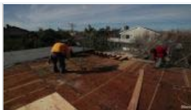
Rebuilding Fire Island
