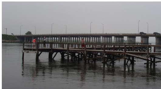
L-Shaped pier at West Marina (Photo courtesy of Malynda Nichol)
