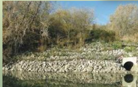
Vegetated Rip Rap
