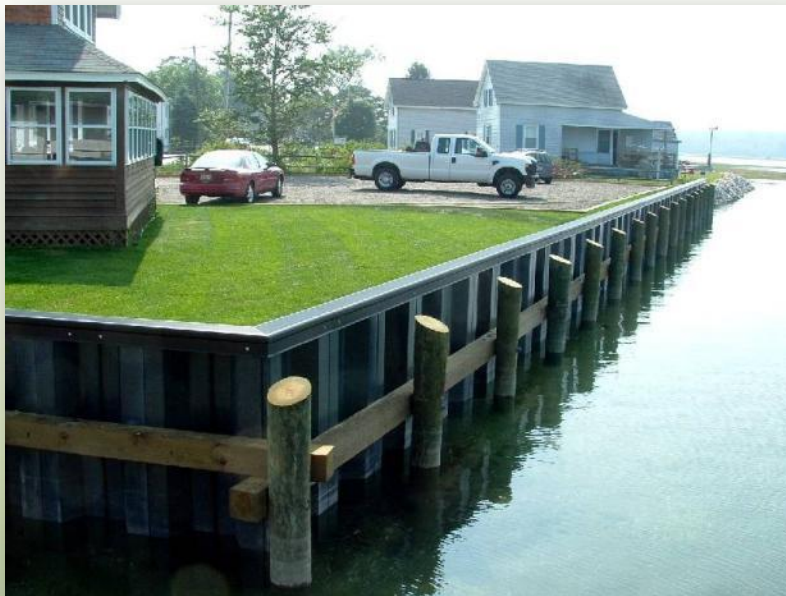
Timber or Sheet Pile Bulkheads
