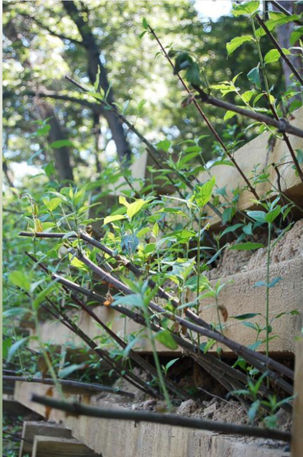
Live Crib Walls
